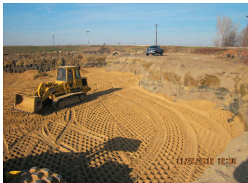
Backfilling after excavation
